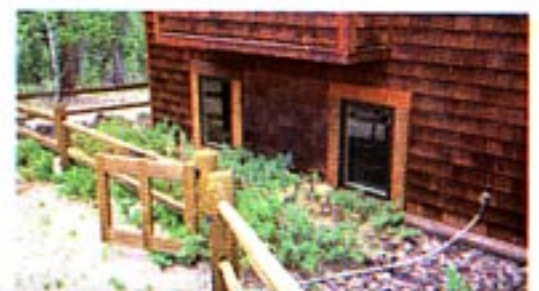
During a wildfire, airborne embers may land and accumulate in the area next to the house. Avoid using combustible materials, such as wood mulch, and flammable plants, such as juniper, within 5 feet of the home.
