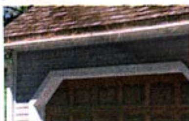
An accumulation of pine needles in rain gutters is a fire hazard. Clean out rain gutters at the start of the fire season.
